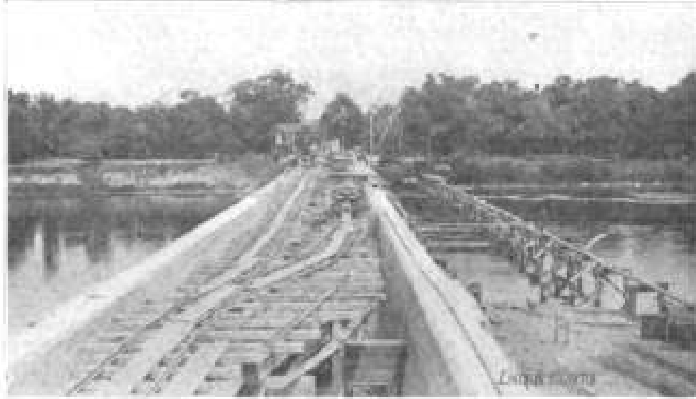
Fig. 2—View Showing Service Tracks and Travelling Derrick Track, Elk Run Bridge.
