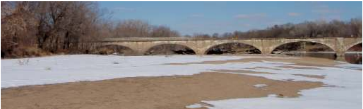
South side of McFarlane Bridge, looking to the North
