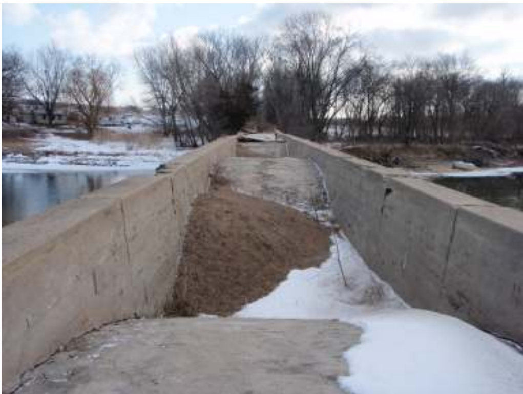
Top side of McFarlane Bridge, looking to ESE
