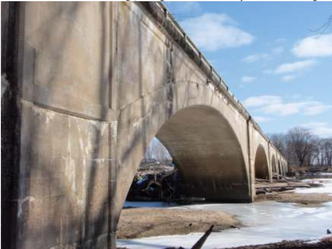
West end of McFarlane Bridge, looking to the East at underneath of bridge
