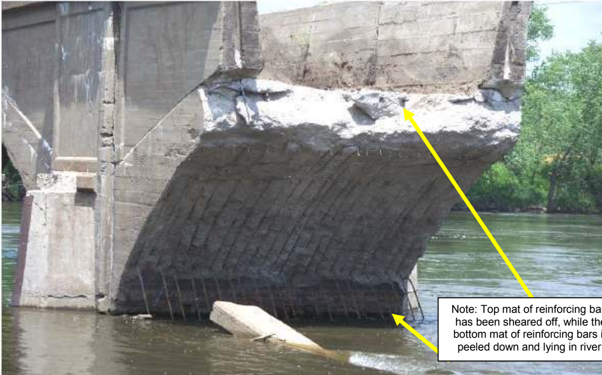
Photograph taken during demolition of Evansdale Bridge showing same type of reinforcement as the McFarlane Bridge. Source: Vern Fish, Black Hawk County Conservation
