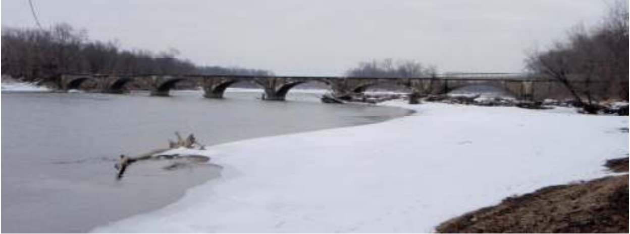
North side of McFarlane Bridge, looking to the SSE
