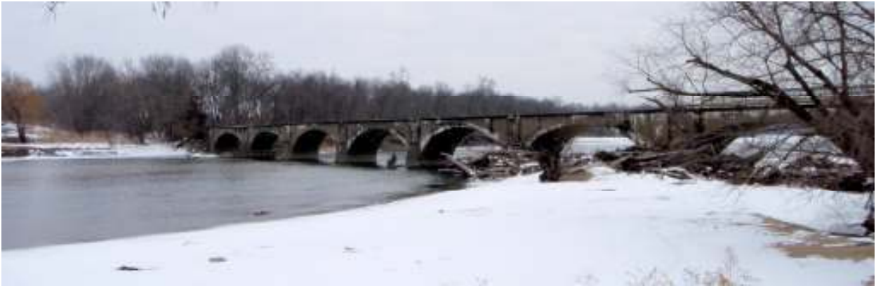
North side of McFarlane Bridge, looking to the SE
