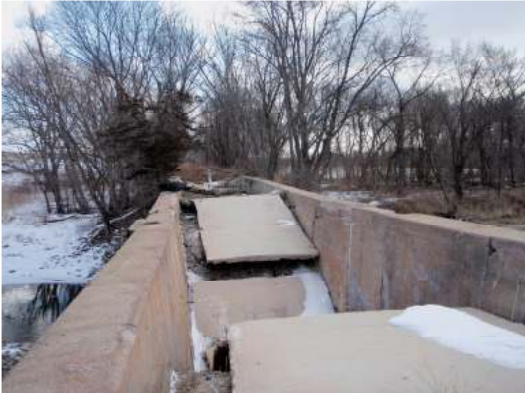
Top side of McFarlane Bridge at east end, looking ESE
