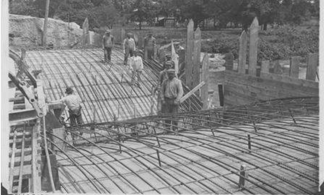
Construction photograph of the Mason City Stewart Avenue Bridge in 1914 showing detail of reinforcing bars and wooden framework prior to the concrete pour of the arches. Source: IDOT Digital Archives, Photo ID HA1.02.0139, accessed at http://historicalphotos.iowadot.gov , March 2012.
