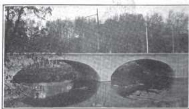
W., C. F. & N. Ry.—Double-Track Concrete Bridge on Cedar Falls Line
