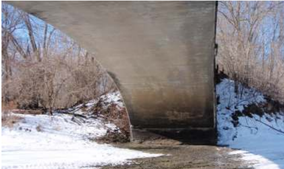
Underside of west end arch of McFarlane Bridge, looking to ENE
