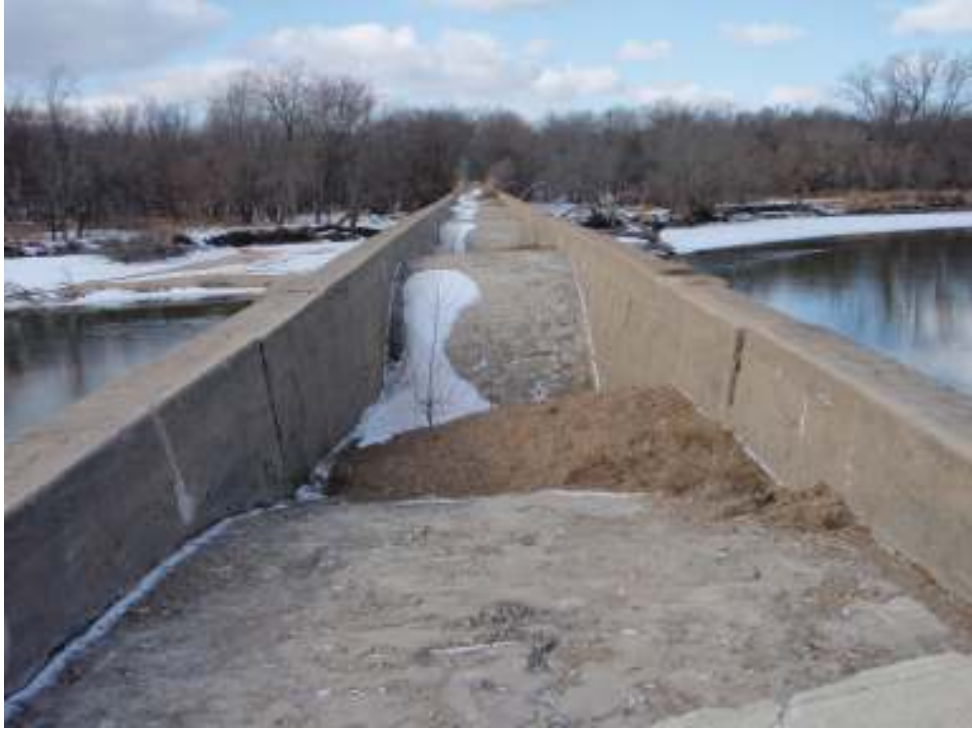
Top side of McFarlane Bridge looking to WNW
