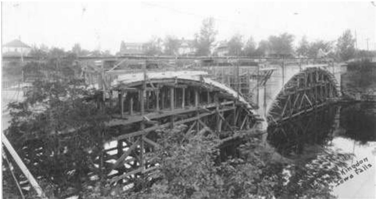
Photograph of arched bridge under construction in Iowa Falls between 1920 and 1930 that shows a side view of the timber framework in place. Source: IDOT Digital Archives, Photo ID HA1.02.0618, accessed at http://historicalphotos.iowadot.gov , March 2012.
