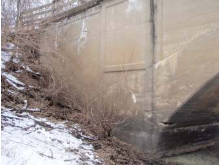
Detail of west end of McFarlane Bridge showing abutment, looking WNW
