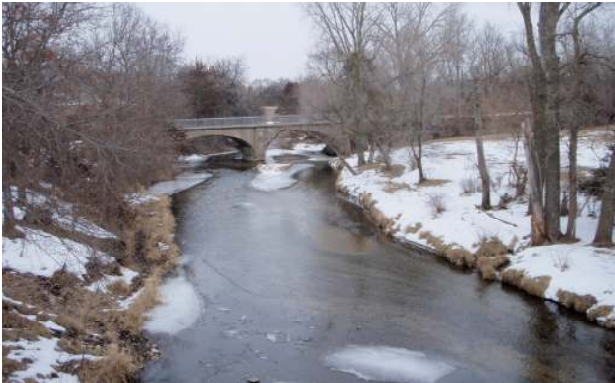
WCF&N concrete arched bridge over Lime Creek just east of Brandon, Iowa. View is looking to the NE from the road bridge downstream of the arched bridge. Field Date: February 9, 2012
