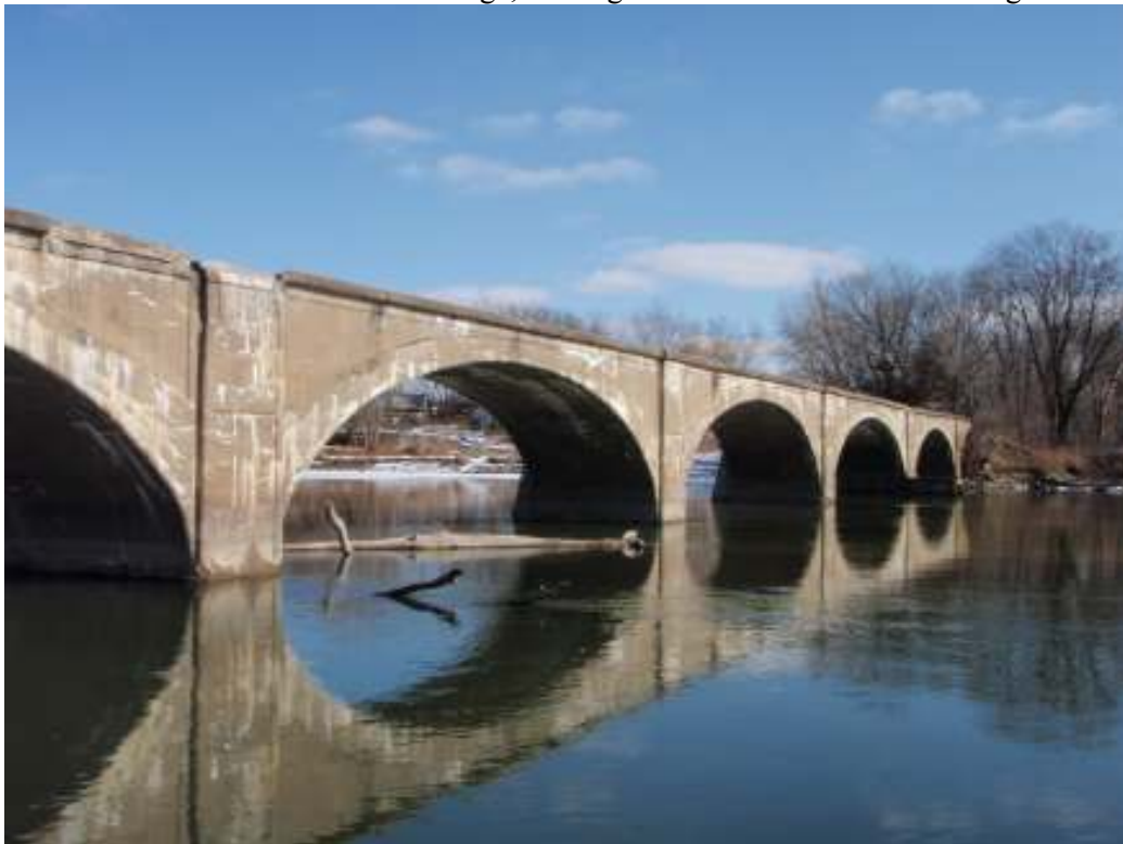
East end of McFarlane Bridge, looking to East
