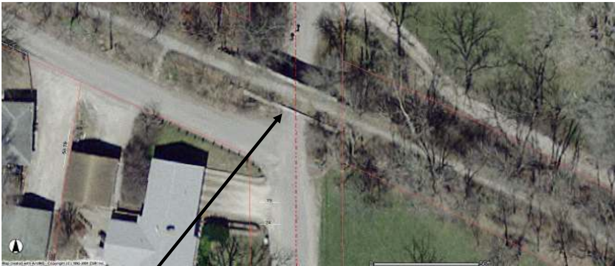
Aerial view of single-arch span over N. Hackett Road in Waterloo, IA. Photograph obtained from Black Hawk County Assessor's Website accessed at http://www2.co.black-hawk.ia.us , May 2012.
