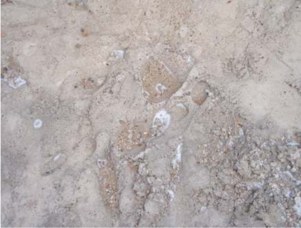
Looking down at bootprints impressed into the surface of the concrete arches during original construction of McFarlane Bridge
